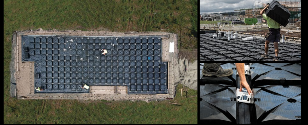
4 X-PODS, KEYSTONE CLIPS, MINI PODS INTO PLACE
