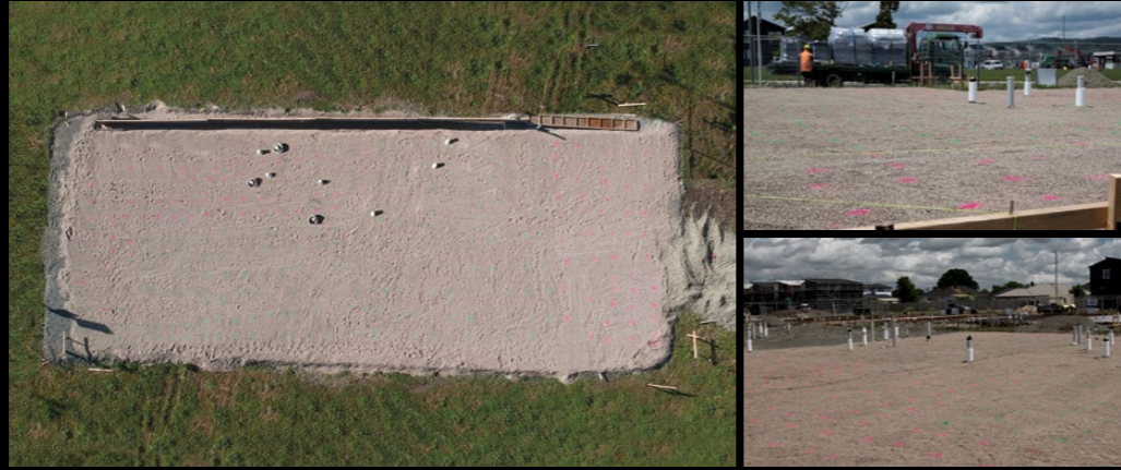
1 SCRAPE AND LEVEL SITE
