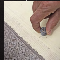
60mm tornado wire screw connectors are placed at 600mm centre intervals to provide regular fixed anchor points into the concrete slab
